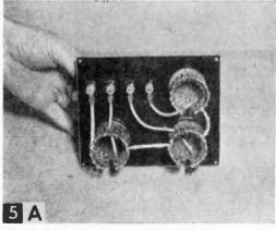
Back of the completely wired unit is shown in A. Use #16 insulated wire from the binding posts and also between the ring terminals.
