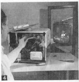
The service tech uses on insulated plastic wond to tap tubes. He watches the screen in a mirror, or reflected from a window. Errotic picture or sound pinpoints the foulty tube.
