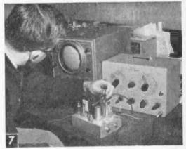
Aligning the converter for the desired VHF band with the aid of a sweep generator and oscilloscope.
